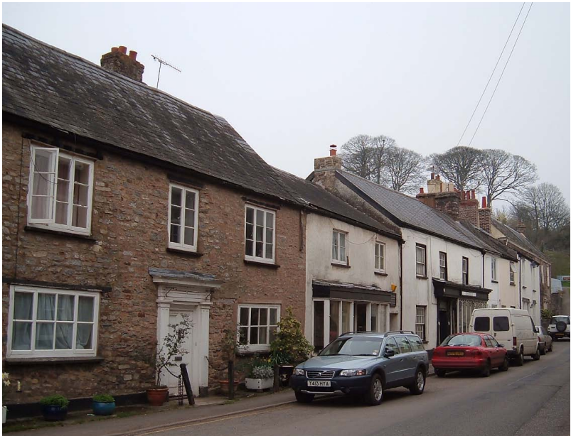
1 Unbroken front roof slopes
