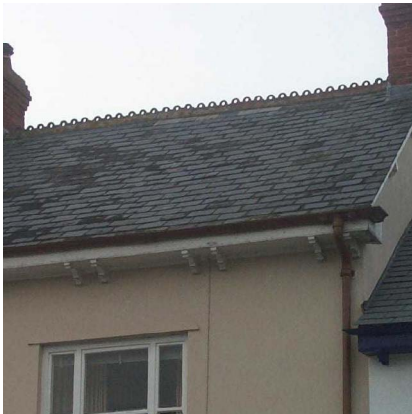
14 Ridge tiles with pierced pattern typical of Bradninch. Plain ridge tile on adjoining property
