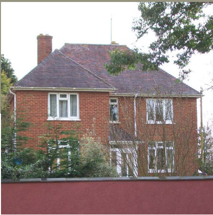
11 Classic hipped roof with covering of red clay tiles
