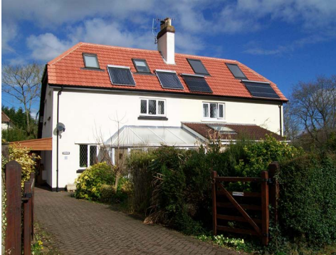
19 Array of rooflights and solar panels
