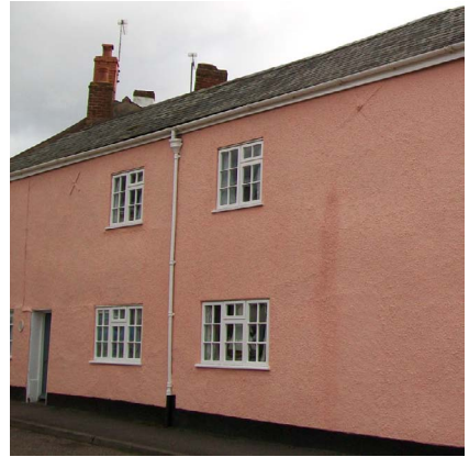
15 Fascia board carrying the gutters
