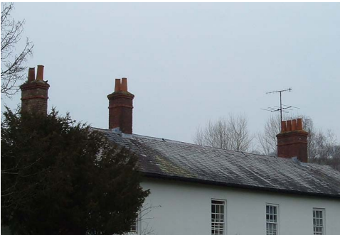
8 Profiled brickstack and matching tall round chimney pots
