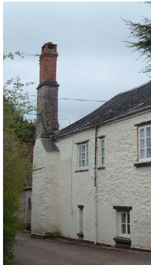
5 Massive external stone stack with brick extension
