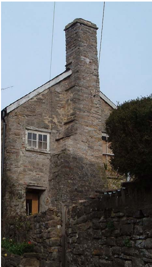
4 Massive external end stack with haunching
