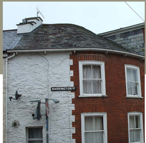
13 Example of curved slating a particular feature in Tiverton
