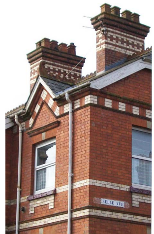
6 Distinctive chimney stack profile with attractive brick pattern and square chimney pots typical in Cullompton
