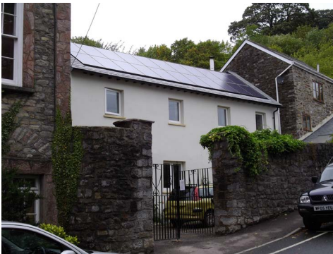
20 Roof covered in PV panels
