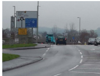
Up-grade Motorway Junction 28 so as to be fit for purpose
