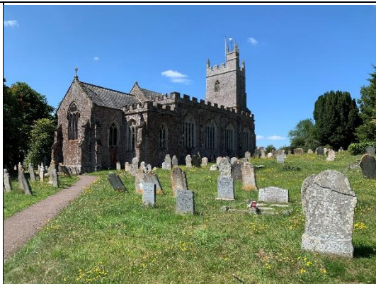
Figure 4.15 Church including tower of St Mary
