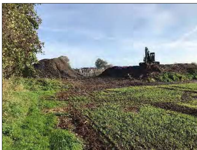
Photograph 5: View of former pond now storage area, looking east
