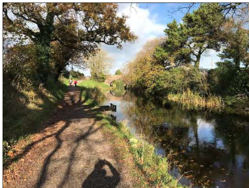
Photograph 7: View along the canal to the Crownhills Bridge (LB3), looking north
