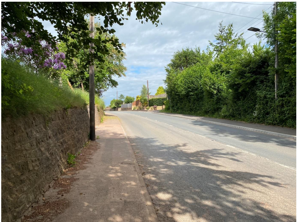
Figure 3.3: Local Pedestrian Facilities
