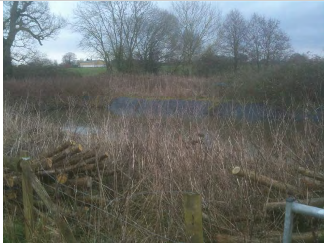
Photograph 6: Plastic-lined slurry pit.
