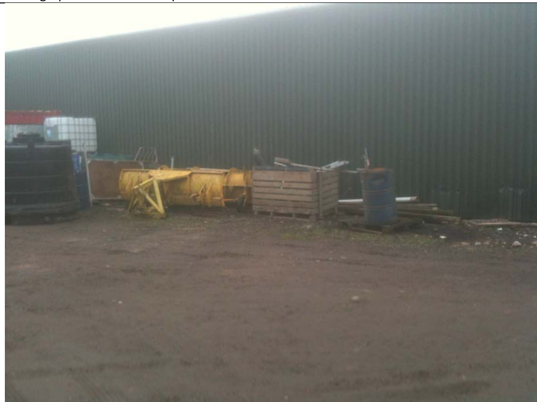
Photograph4: Mixed storage with minor oil spill.
