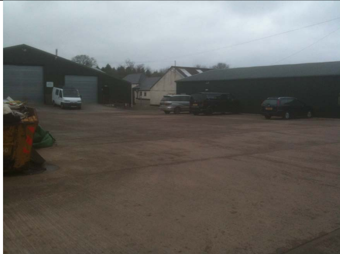
Photograph 5: The more modern steel framed business warehouses.
