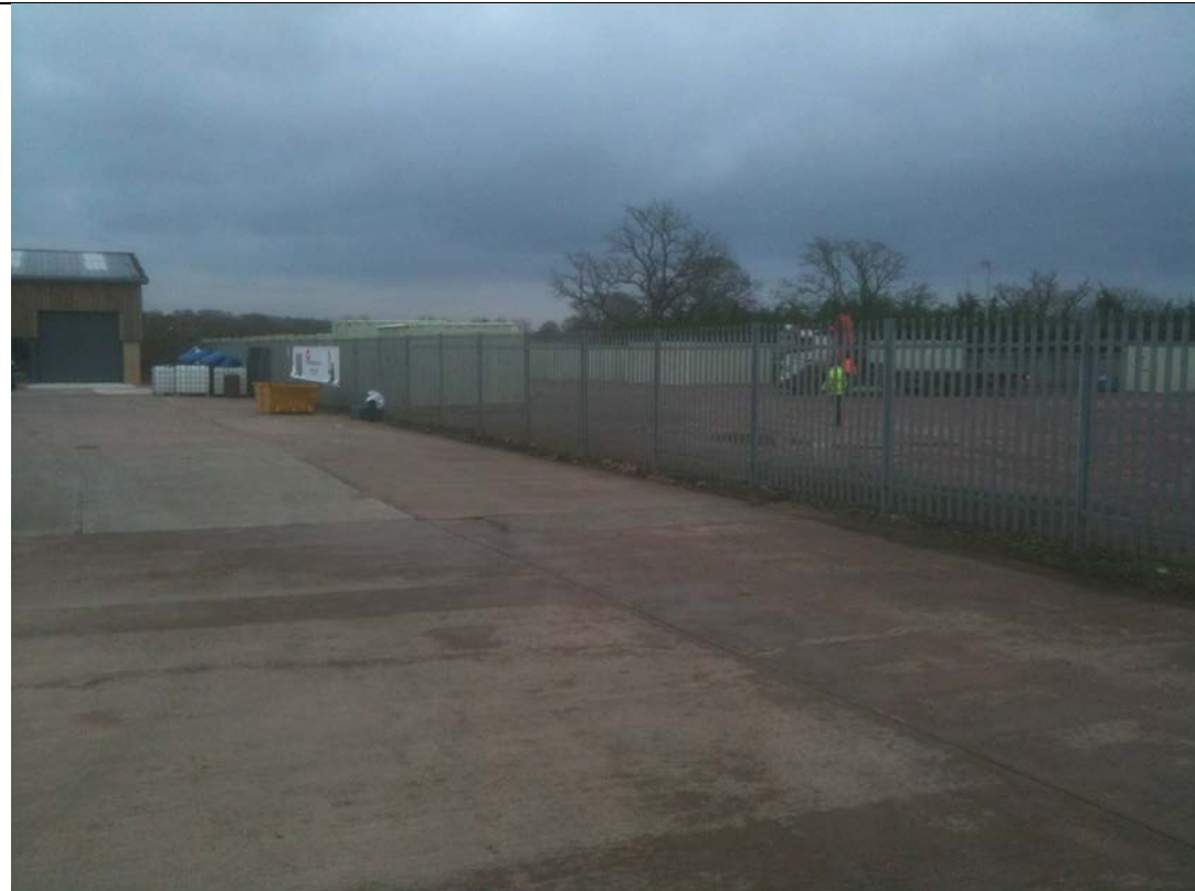
Photograph3: Plant hire compound
