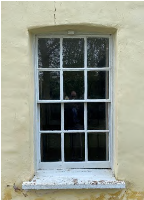
Timber sash window upon Moorings
