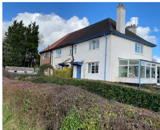
Quarry View Cottages
