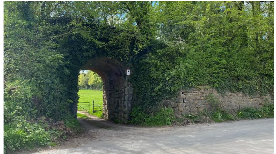
Surviving stone archway for the Westleigh Mineral Railway
