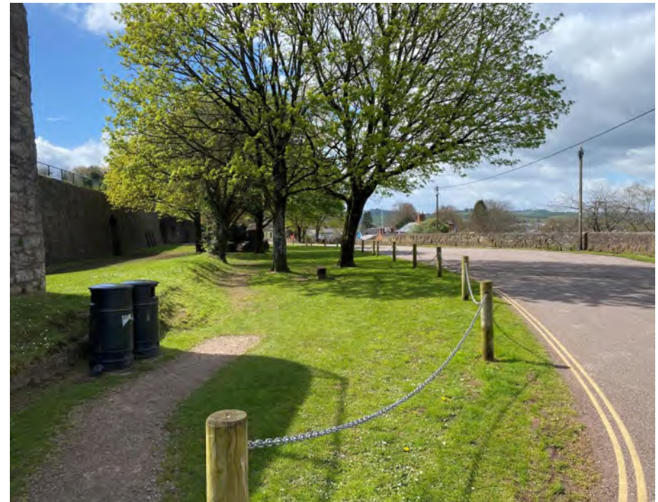
View of entrance to the canal within Tiverton with lime kilns to left hand side
