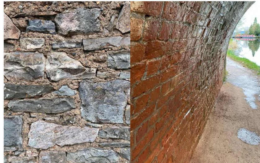
Left, stone walling, right English bond brickwork
