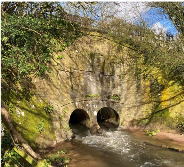
Grade II listed Twin Culverts for the Grand Western Canal
