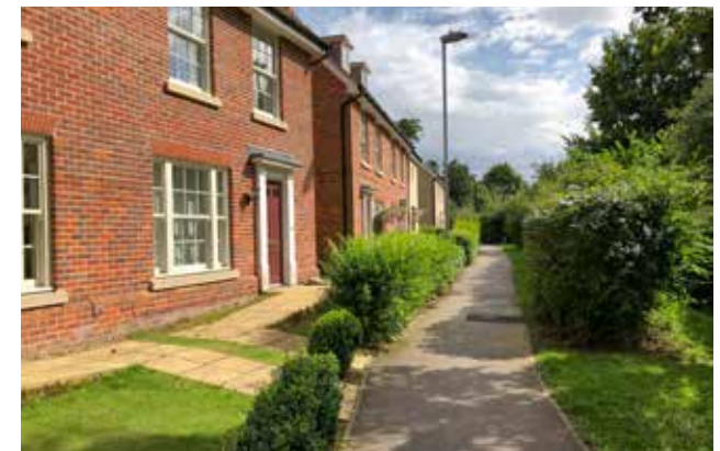
Fig.49 Precedent: Saxmundham, Suffolk The successful integration of existing green infrastructure such as hedgerows, trees and green spaces which are fronted by new homes
