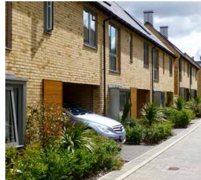
Fig.41 Examples of integrated and attached garages
