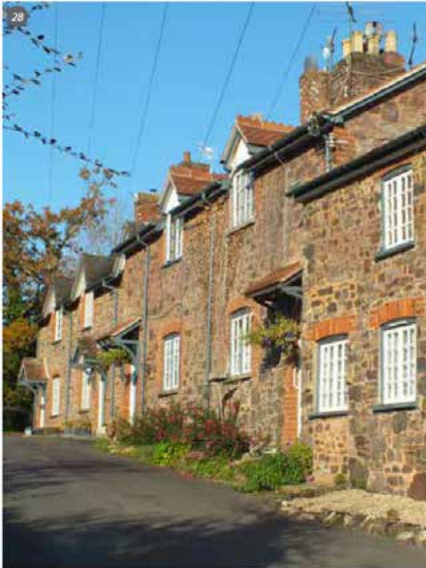
Fig.19 local architectural character
