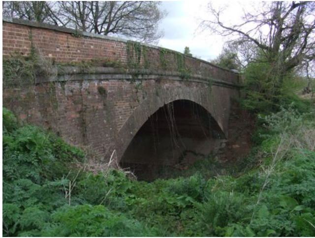
Plate 7: Manley Railway Bridge
